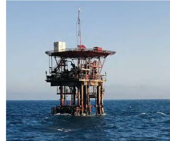
Platform with DSL Rigged Up
