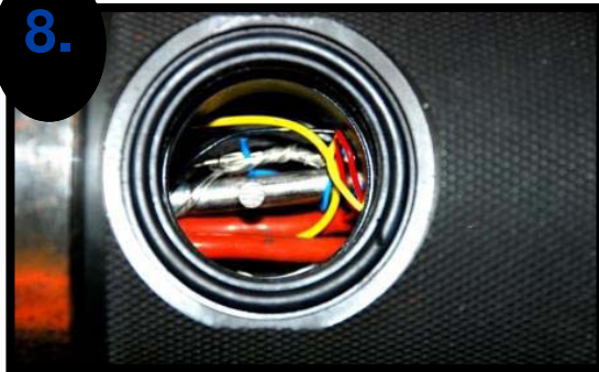
Inspect wiring, remove shunt
